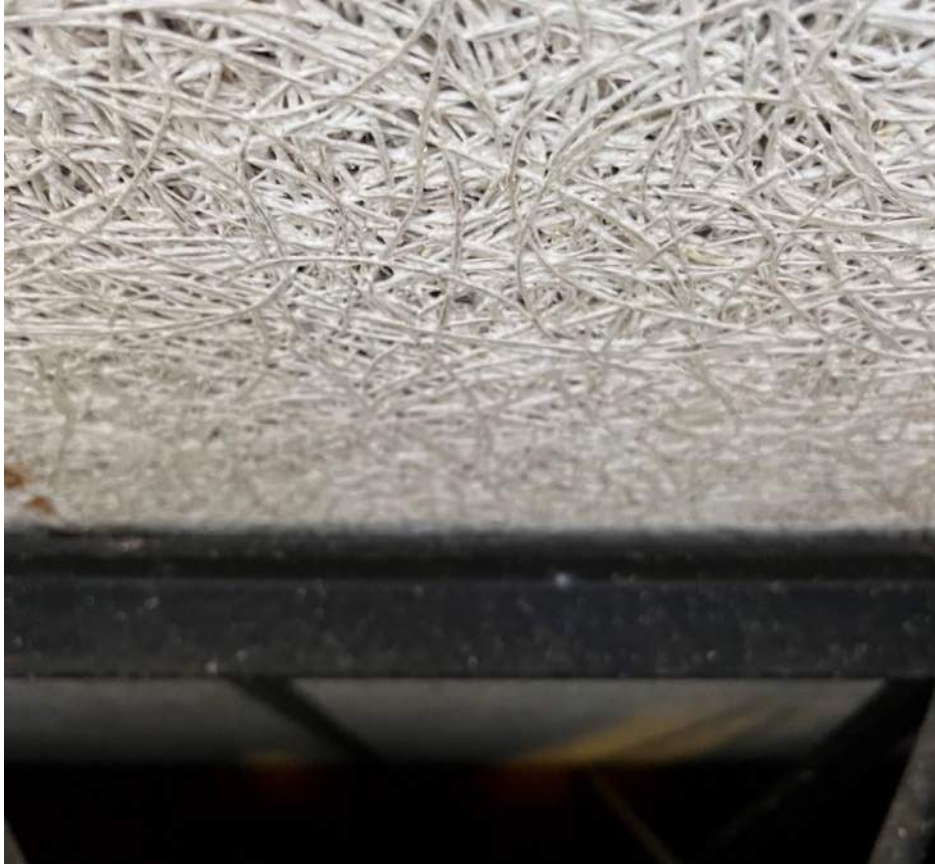
Tectum Decking on the Original West Roof Area
