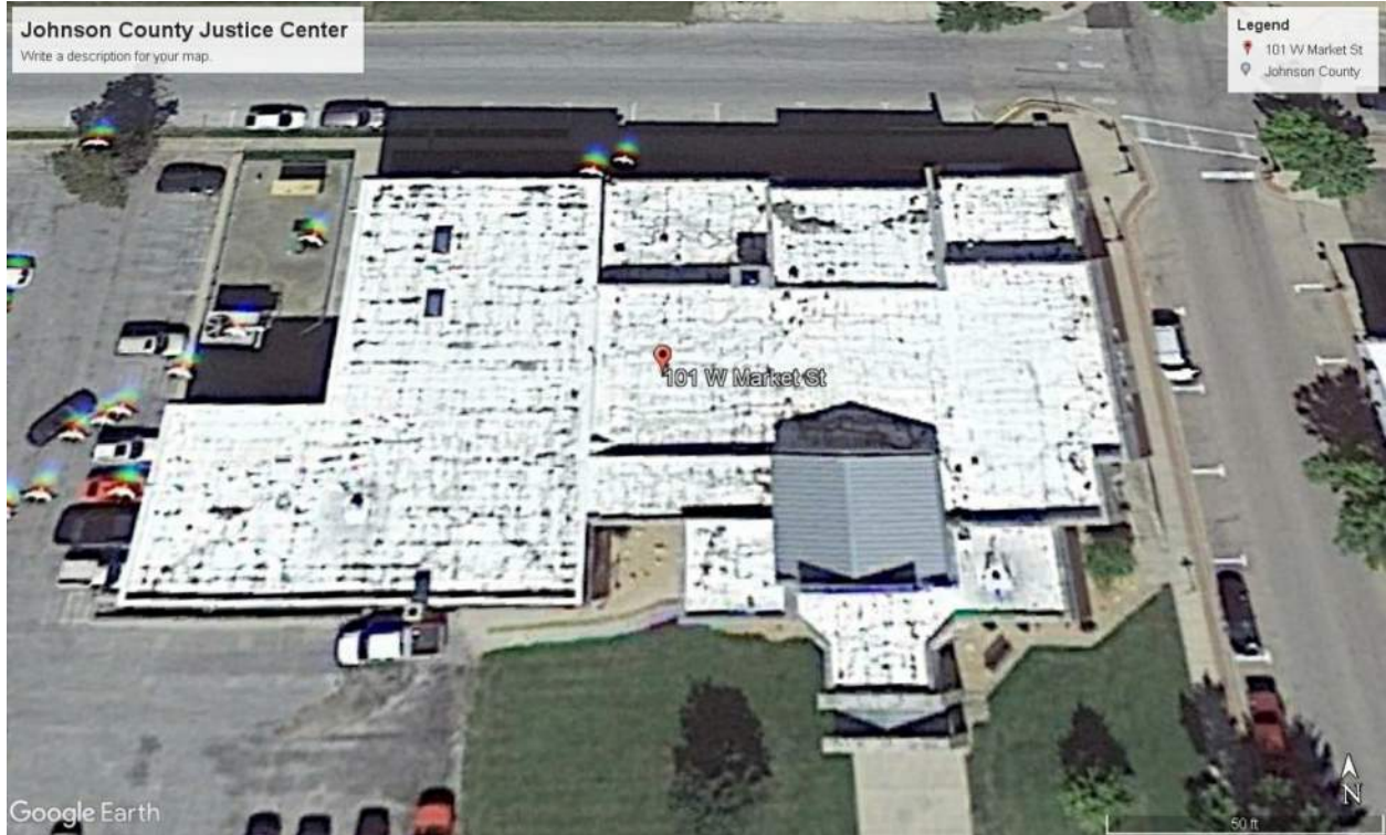
Johnson County Justice Center Roof Overview
